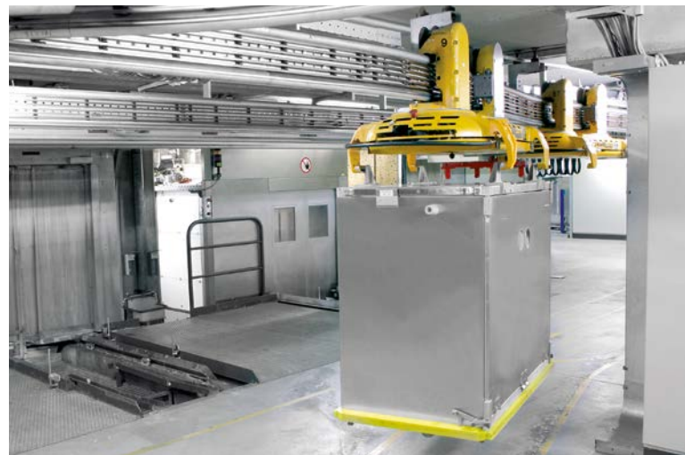
Electrical overhead track
